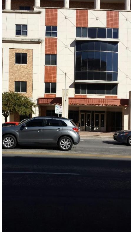
(b) High Point at Student Services Building
