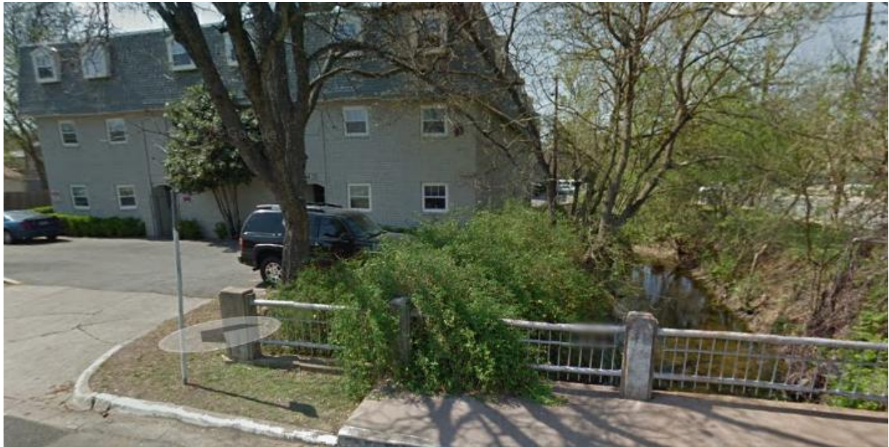
Figure 2: Apartment/Condo Complex (Left) and Waller Creek (Right) along Avenue F
