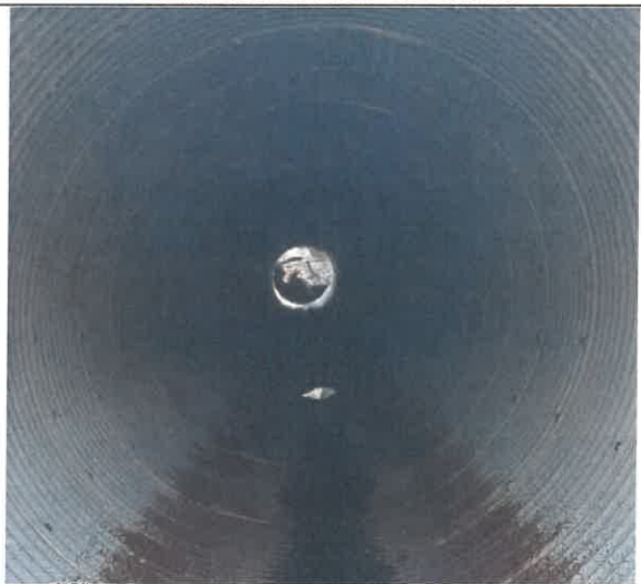
Culvert Pipe under the road (4 ft diameter)
