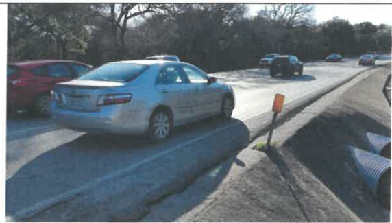
Downstream view of culvert
