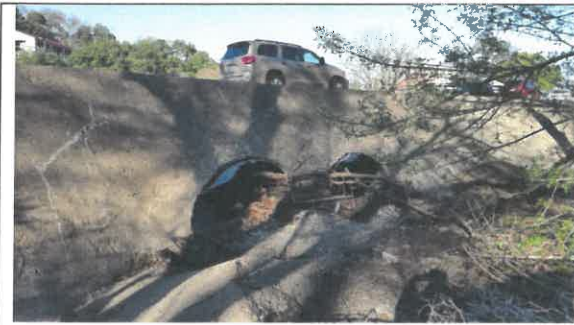
Upstream view of culvert
