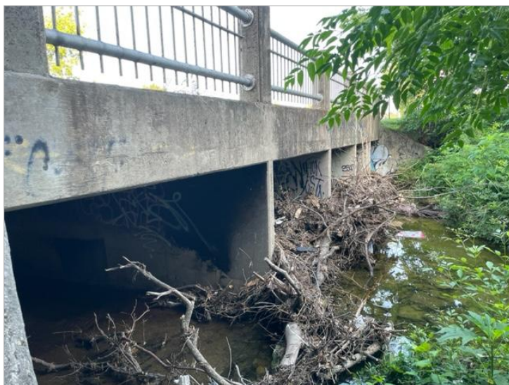
Figure 18. Upstream view of Shoal Creek at Anderson Lane stream crossing.
