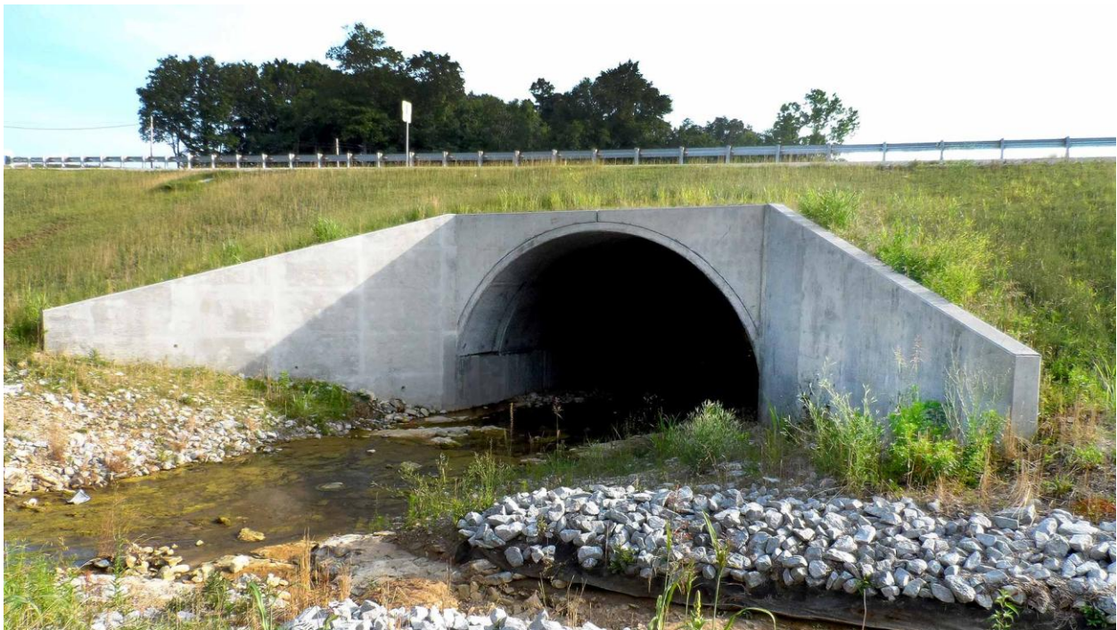
Figure 2. Arch Culvert Example 1.
