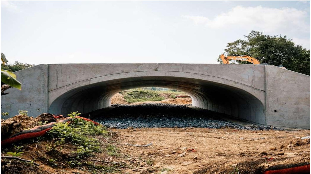
Figure 3. Arch Culvert Example 2.
