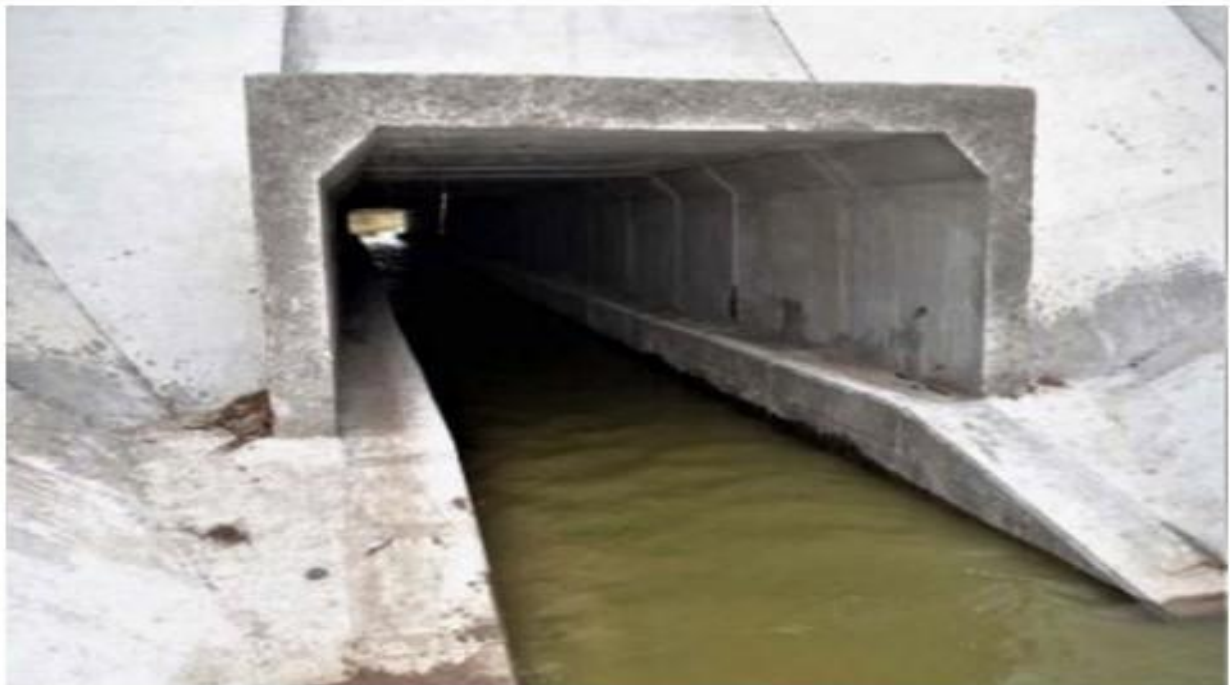
Figure 4. Culvert with ledges for animal passage.
