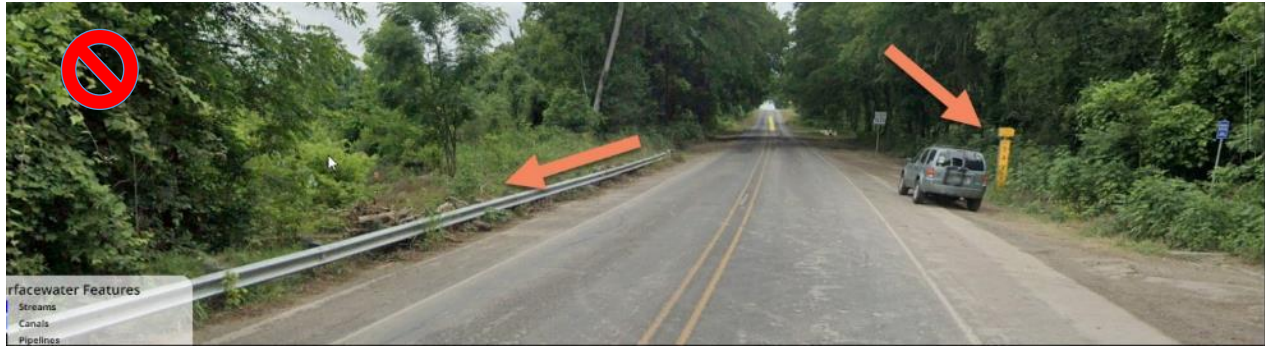
Figure 4.4. Example of a bridge with flood debris and a depth gauge.
