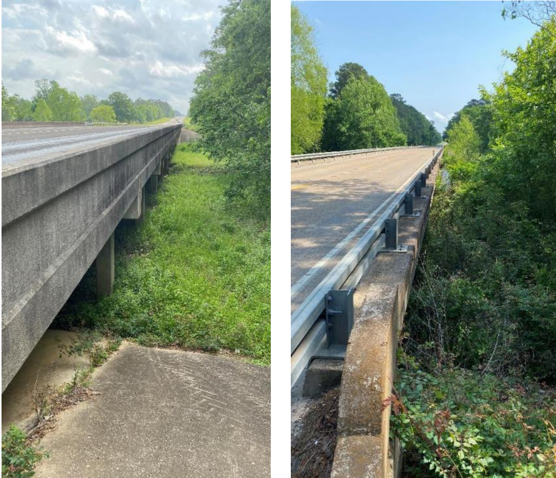
Figure 4.8. Example of clear (preferred) vs. overgrown cross section (not preferred).
