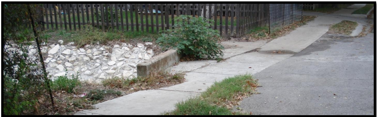
Figure 5. Street runoff enters creek directly
